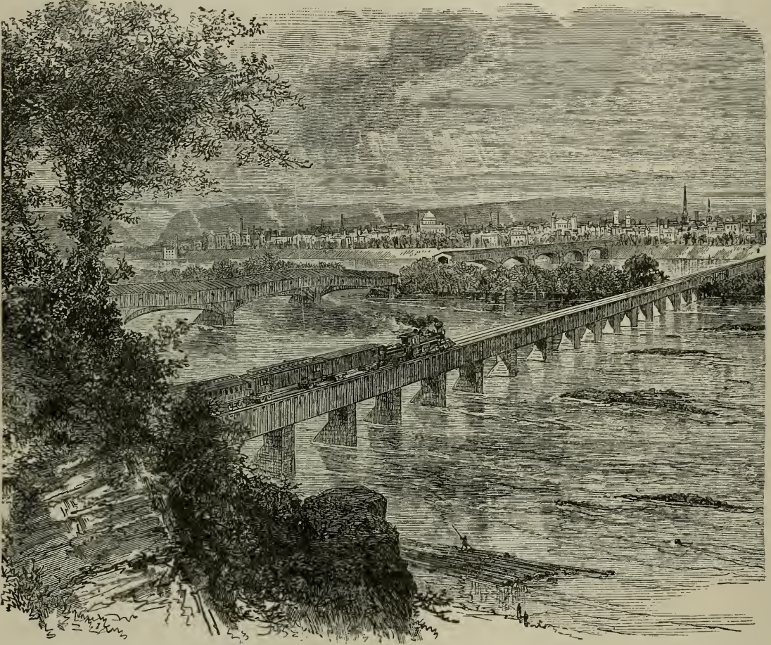
BRIDGE CROSSING THE SUSQUEHANNA RIVER AT HARRISBURG.
